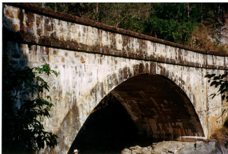
Historic Little Crystal Creek Bridge
