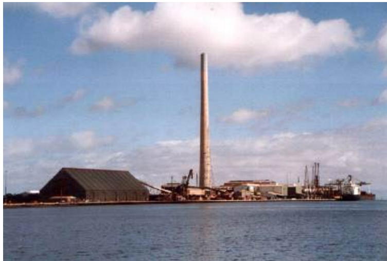
Smelter at Port Pirie
