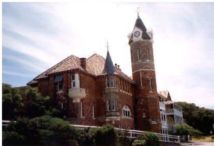
Old Post Office - Albany
