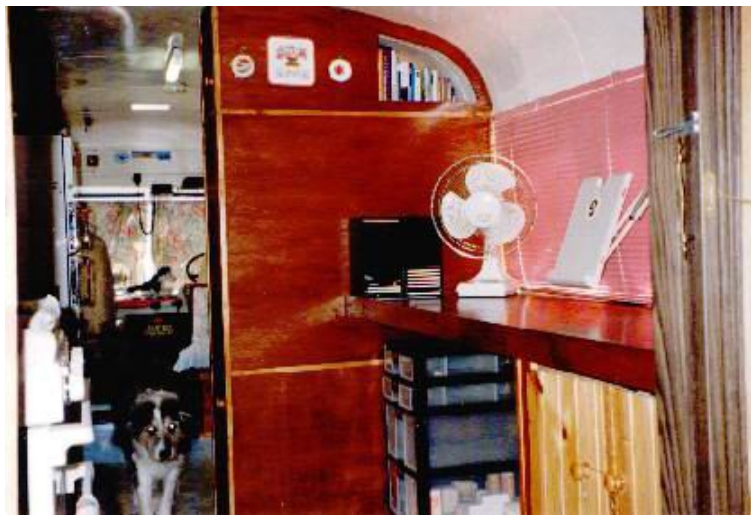
New cabinet work
