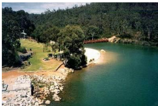
North Dandalup Dam
