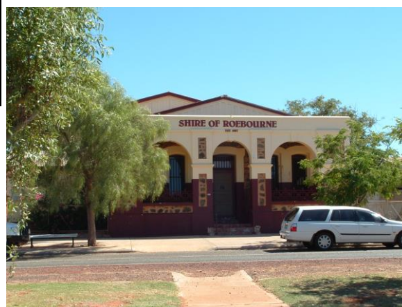
This used to be the Union Bank
